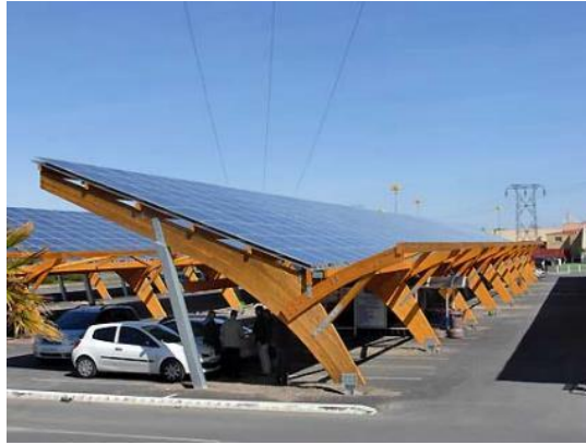
Figure 78 : Ombrière photovoltaïque
